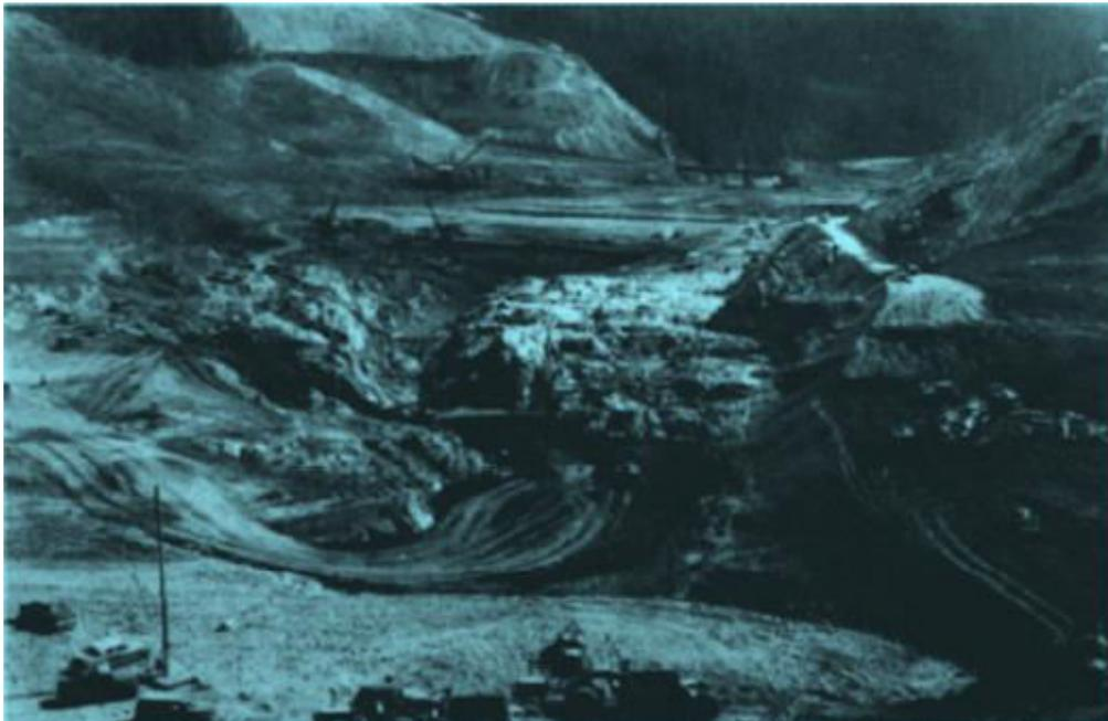
Figure 18. Excavation for Tawa River dam, showing inner bedrock channel trending along..
