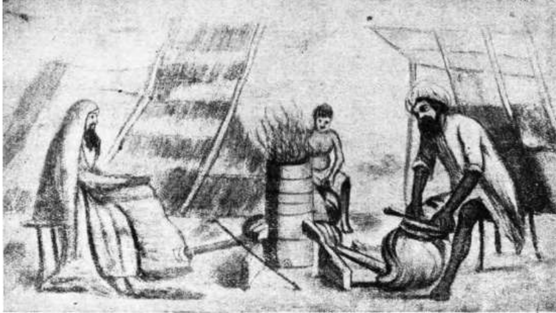
Indian blast furnace for smelting copper (Ball's Economic Geology of India).
