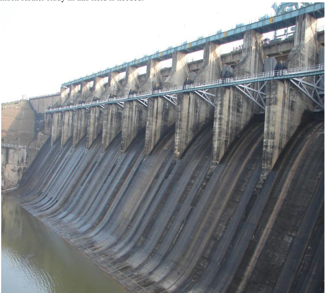
Tawa Dam on the Tawa River.
