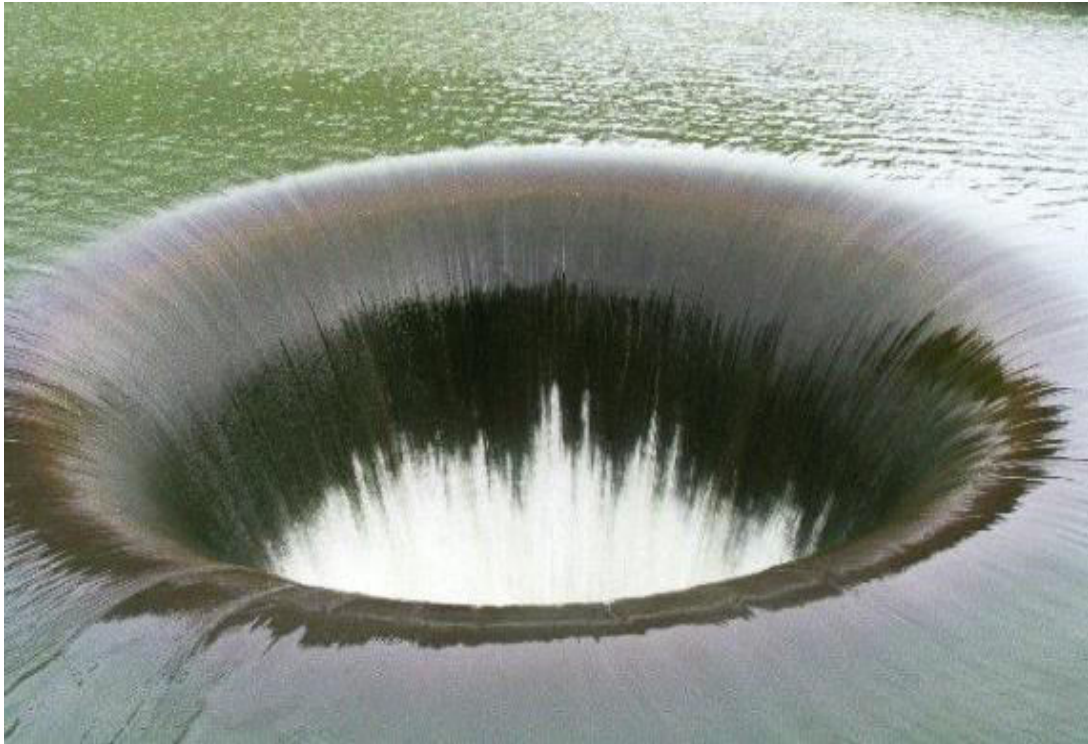
The Monticello Dam in California, United States is most noted for its large circular spillway with a rate of 48,400 cubic feet per second.
