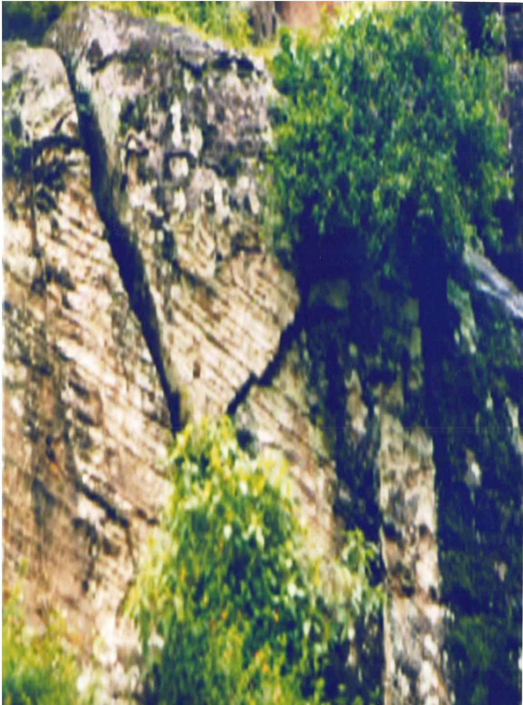
Figure: 23. The consequence of thrust or shear and differ from the commonly accepted thrust planes in that the fracturing is more nearly vertical than horizontal and the direction is more nearly parallel than at right angle to the direction of shear or thrust.
